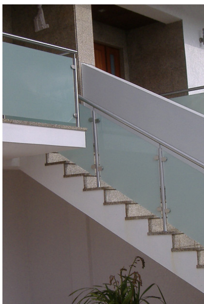
MORADIA UNIFAMILIAR, 2008 Lourosa, Portugal
